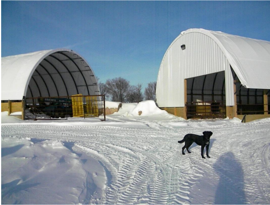
Secondary hoop barn to store manure during winter from scraped alley in 200 head facility
