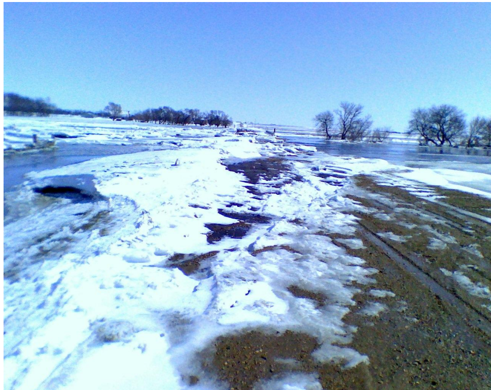
Big Sioux River below Stray Horse Creek flowing over county highway
