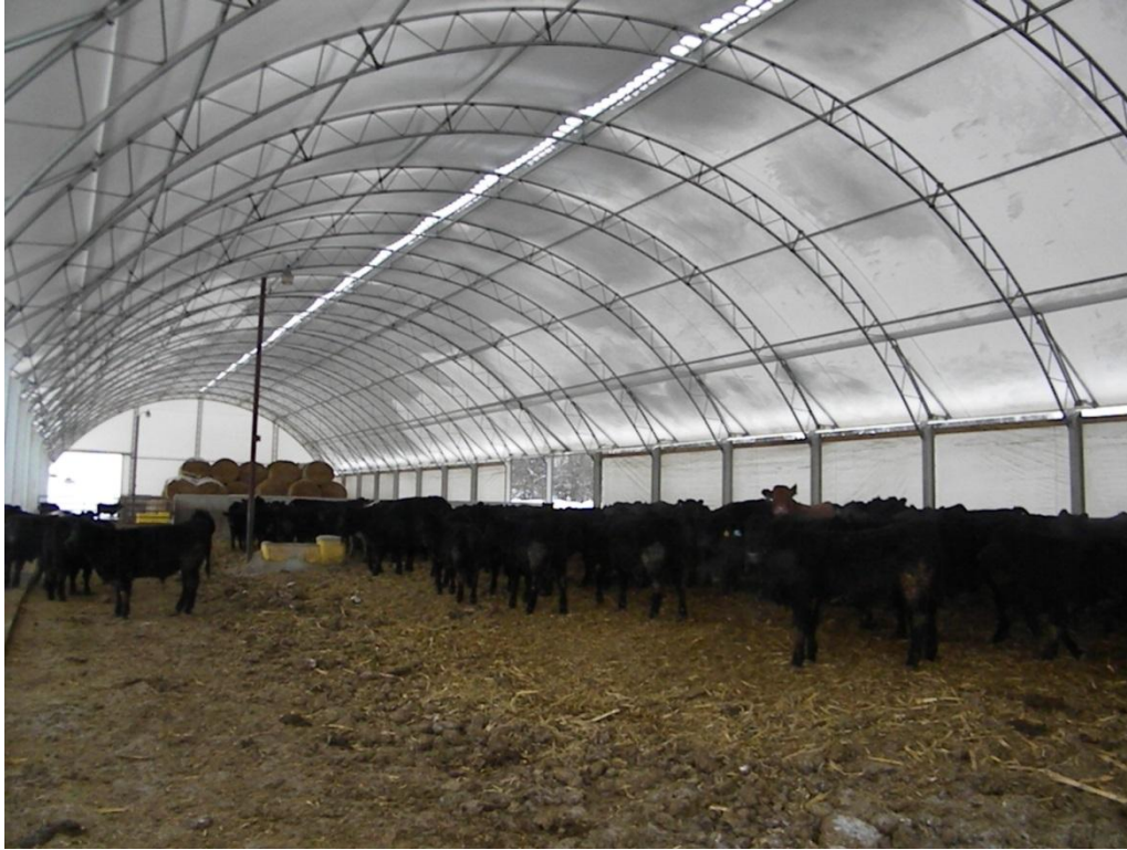
Snow on roof and wet outside, but 400 head facility keeps livestock and manure confined
