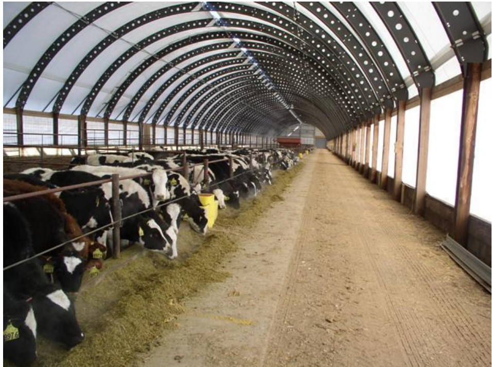
Hoop barn using compost method with inside feeding alley for replacement dairy heifers
