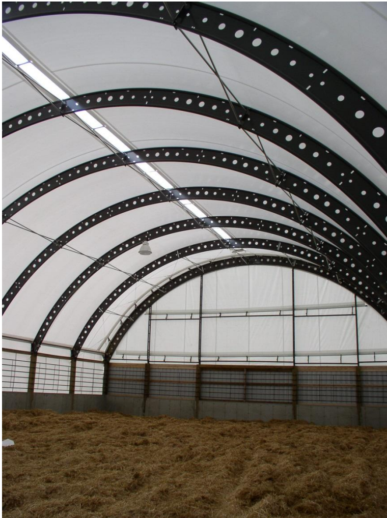
Inside dairy composting barn
